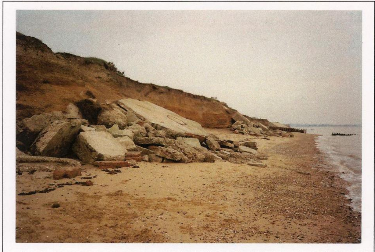
SMR 10030/31: Before coastal erosion caused their demise, the two 4.7-inch gun casemates at East Mersea stood on the cliff edge. They were of the same pattern as the surviving casemate, the 'Two Sugars' at West Mersea. (See photo page 7).
