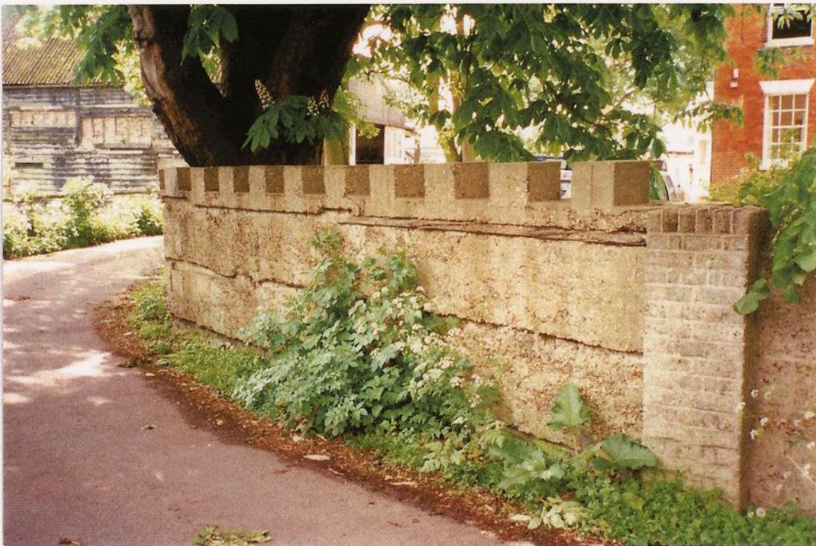
SMR 10894: Documented in wartime records as a 'concrete firing post', this crenellated wall still stands around the garden of Eastbay House, Colchester. From here, infantrymen could fire on to East Bridge, which it overlooks. To camouflage the position, fencing would have been nailed to the horizontal battens.
