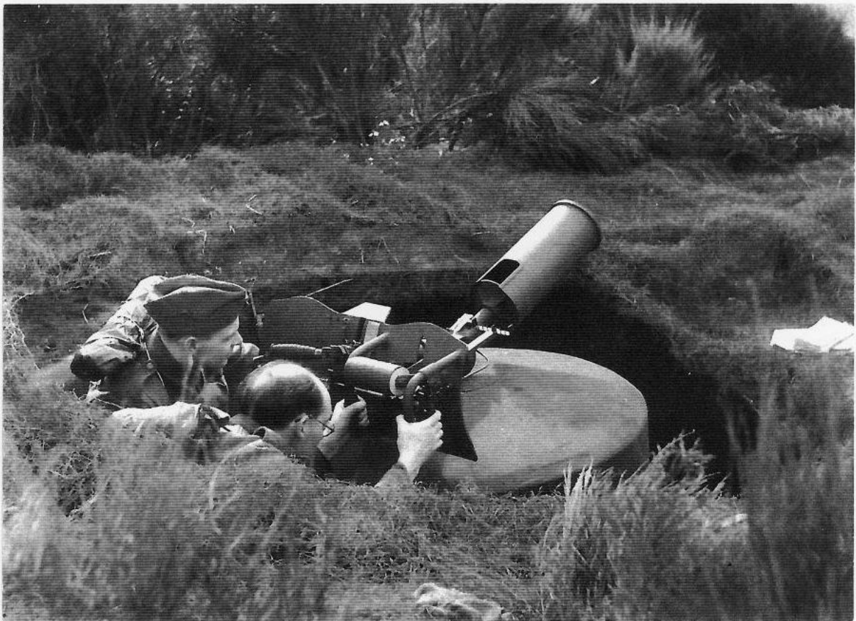
August 1942: Men of Colchester Home Guard on Exercise 'Crack', here manning a 29mm spigot mortar mounted on its concrete pedestal in its purpose-designed pit. (Photograph courtesy of the Imperial War Museum, London. H22518).
