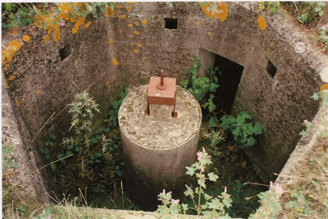
SMR 10958: There are many pillboxes along the Eastern Command Line which feature an anti-aircraft machine-gun well. The weapon, probably a Lewis gun from the First World War, would have been mounted on the central steel pin.
