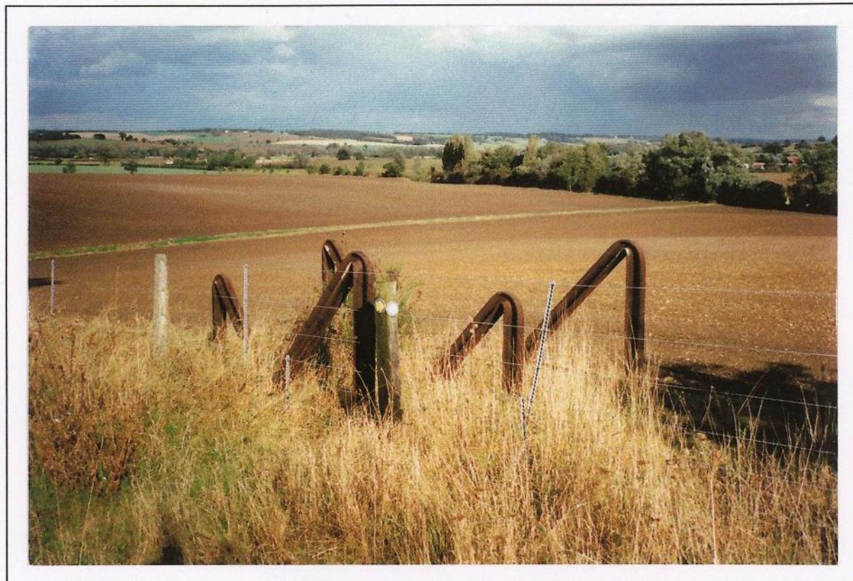
SMR 20030: 'Hairpins' were a common anti-tank device. They were formed from lengths of railway line, cut and bent on site and then either concreted into the ground or dropped into steel sockets. Since World War Two very few have escaped the scrap iron dealer but these, documented in wartime records, still stand at Mount Bures.
