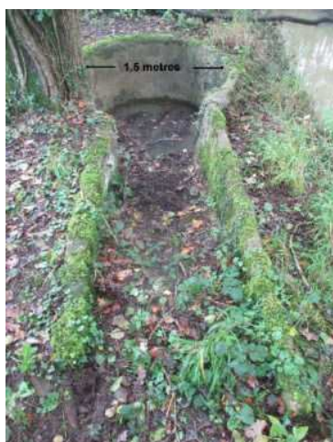
The structure in Birch Woods
