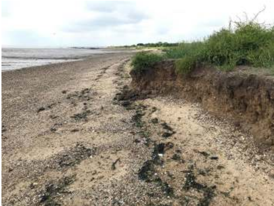
Figure 7. Eastern extent of ramparts looking south. Note the strandline marked by seaweed now cuts through the structure
