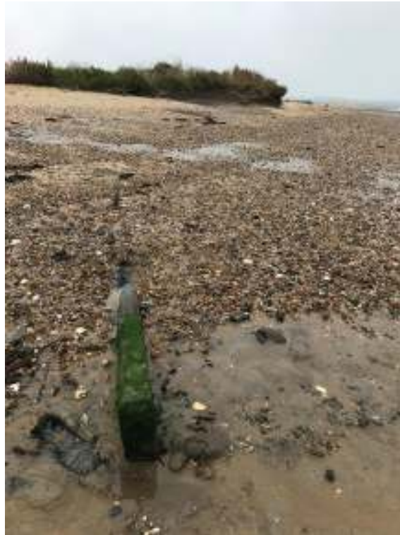
Figure 6. Feature 105 facing due north - a large timber beam in situ with the blockhouse ramparts behind
