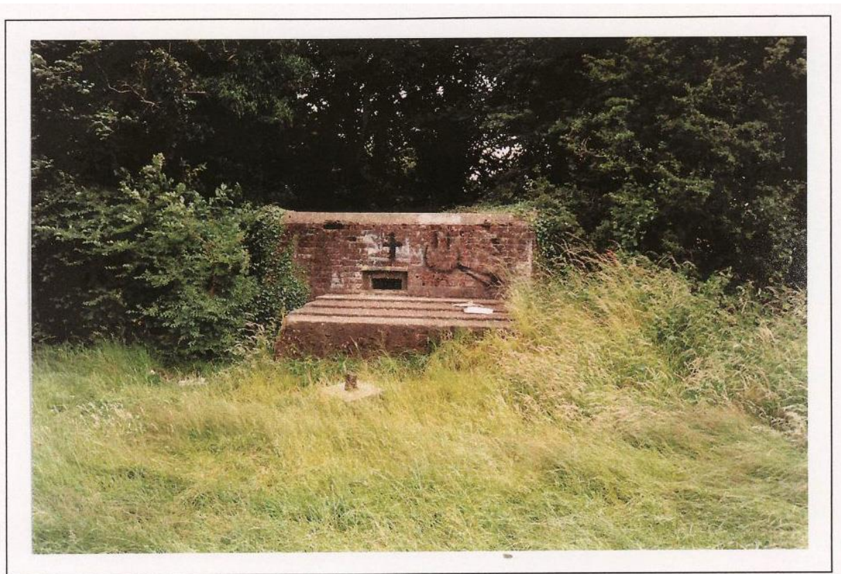
SMR 20614: Pillboxes were designated as 'bullet-proof', generally with 15" walls, or 'shell-proof' with much thicker walls, as with this example.
