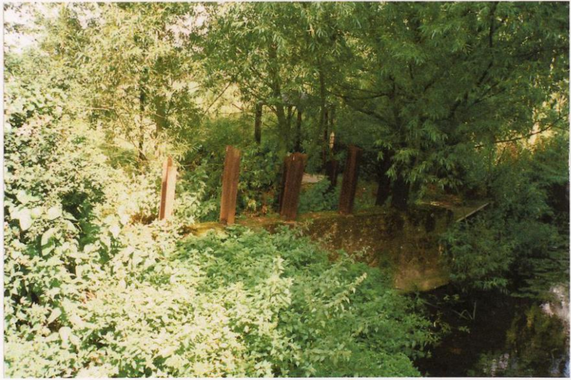
SMR 10939: During World War Two, hundreds of anti-tank rails were concreted into the banks of the River Colne in places where it was thought that armour might be able to cross. All, except these, have fallen beneath the oxy-acetylene cutter.
