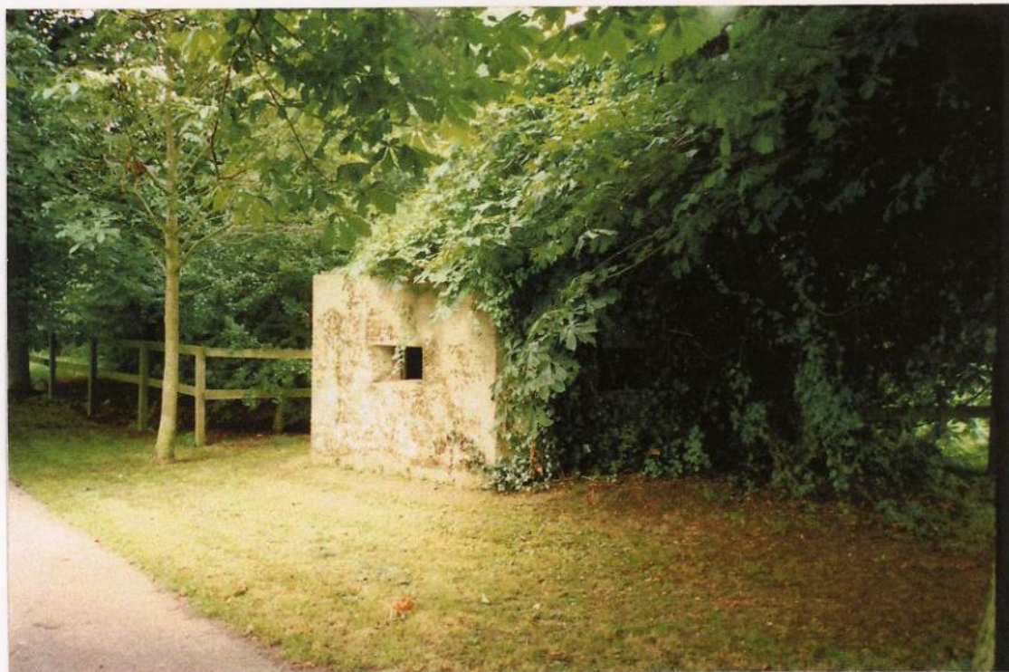
SMR 10960: The FW3/22 was one of the smallest of the pillbox designs during World War Two. Its 15-inch walls were intended to be bullet-proof rather than shell-proof.
