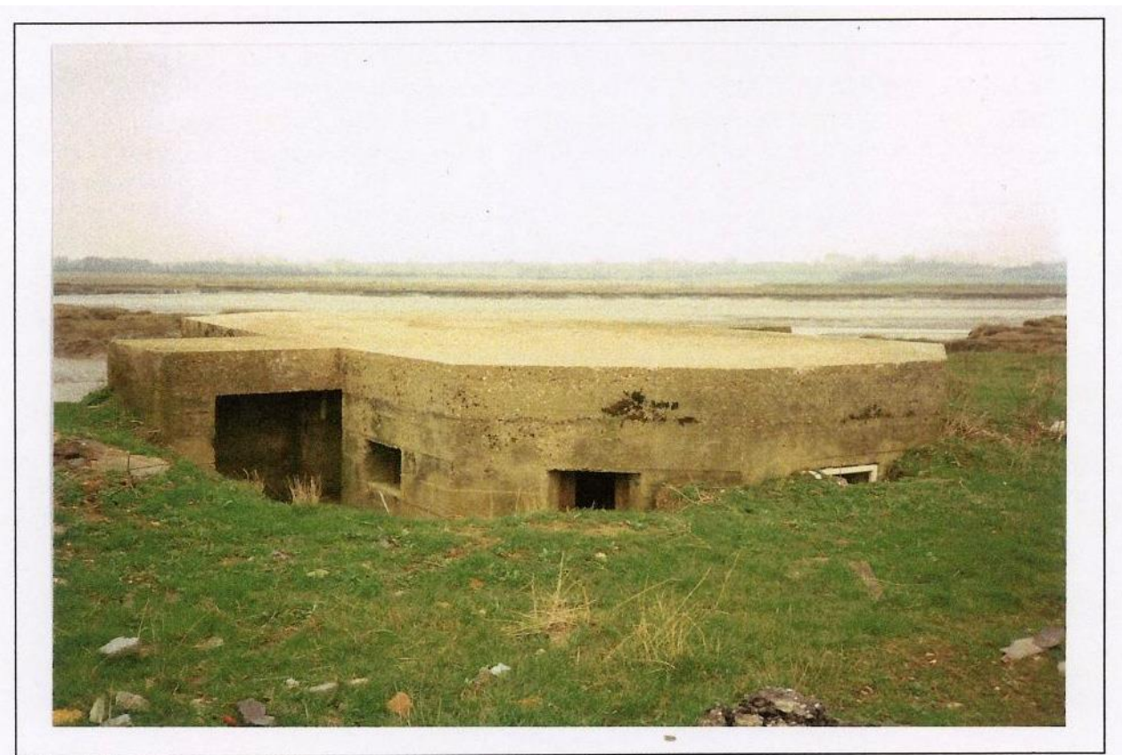
SMR 10043: Although the seawall has been built up, the entrance and loopholes are still clear on this double-ended pillbox.
