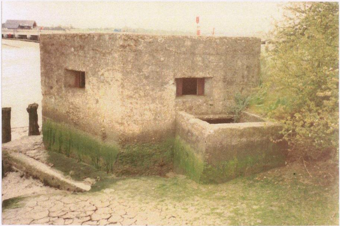
SMR 10877: The picturesque setting of this pillbox somewhat belies its more serious purpose. The drop-in entrance is very unusual; clearly designed to protect against flooding.
