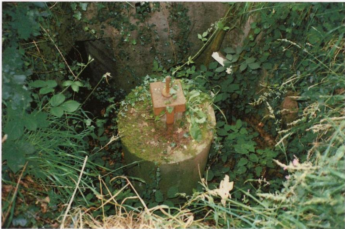
SMR 10945: The central well of the pillbox at Seven Arches Farm. The pedestal, with its steel mounting rod, would probably have held a Lewis gun from the First World War.
