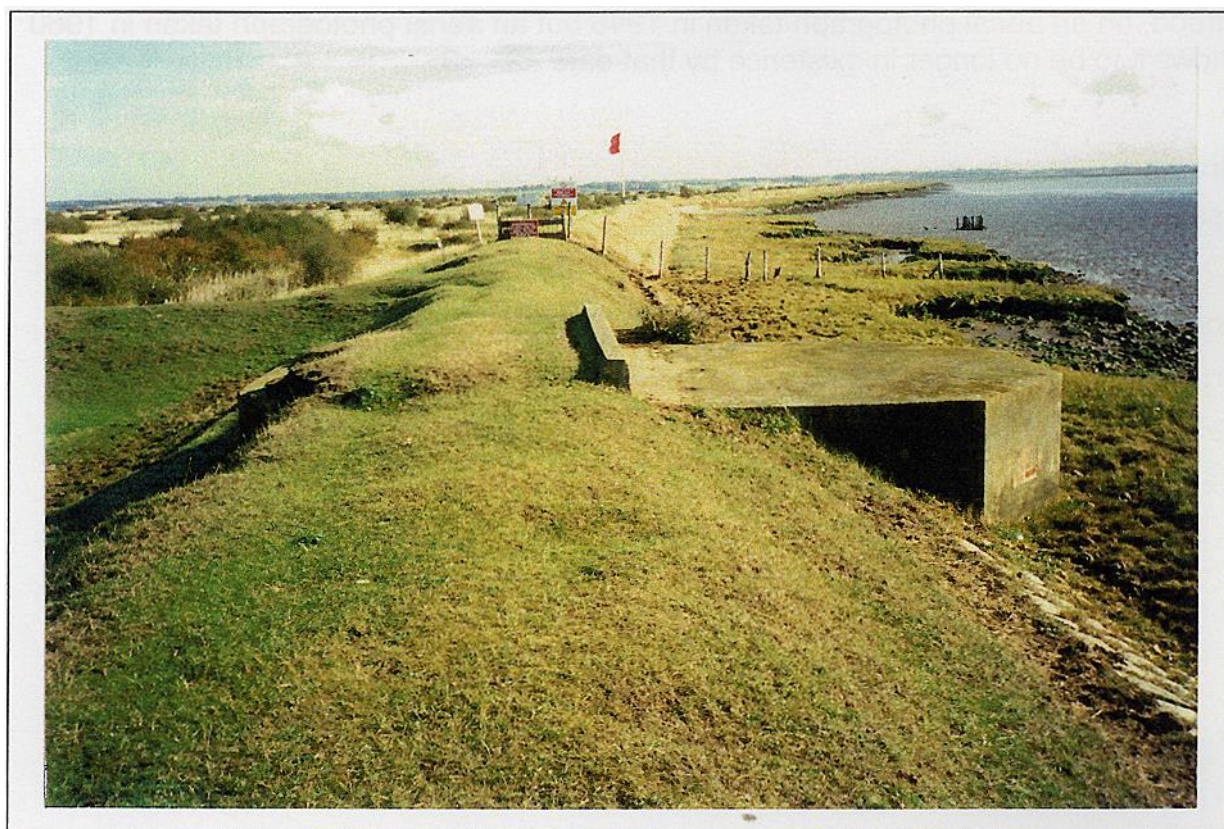
SMR 10732: One of a number of double-ended pillboxes built across the seawall at Langenhoe
