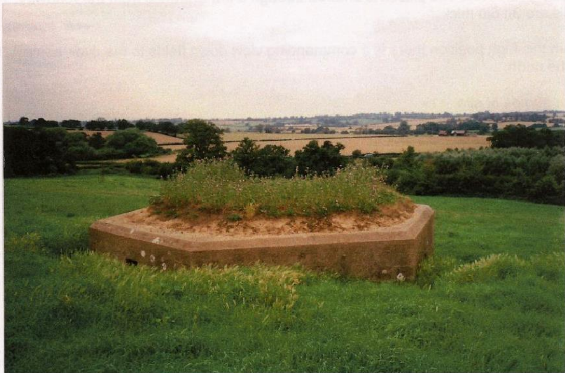
SMR 10958: Earth and grass on top of a pillbox is not a natural result of wind and weather but was a deliberate attempt, at the time of construction, to camouflage it against air attack.
