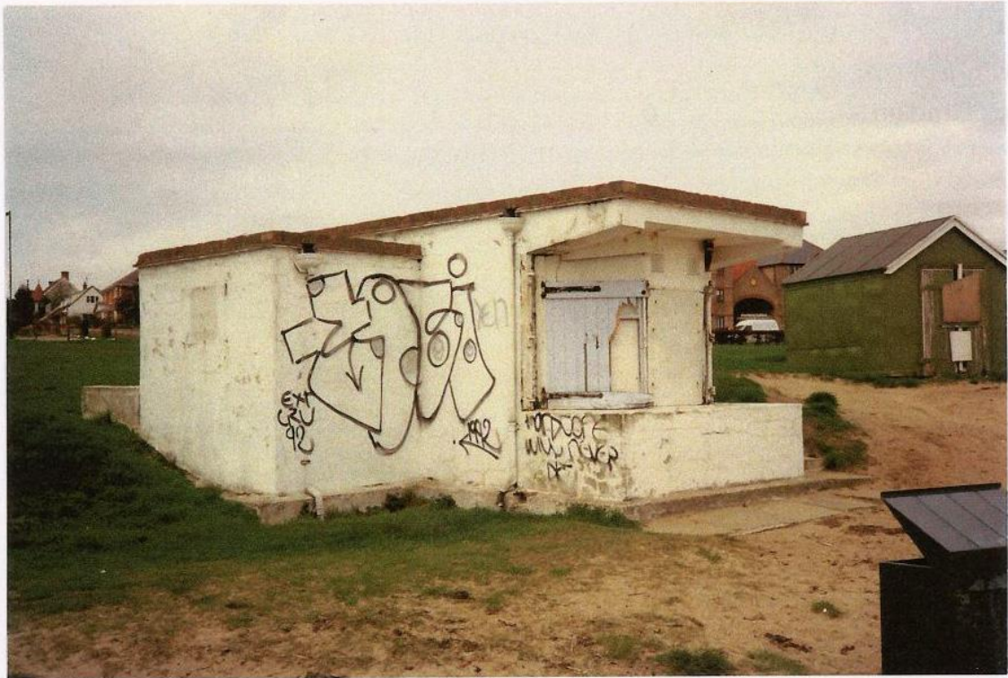
SMR 10041: Only a handful of Coastal Artillery Searchlight Emplacements survive in Essex. This one, at West Mersea, provided the night-time illumination for the 4.7-inch guns (SMRs 10038 & 10039) nearby.
