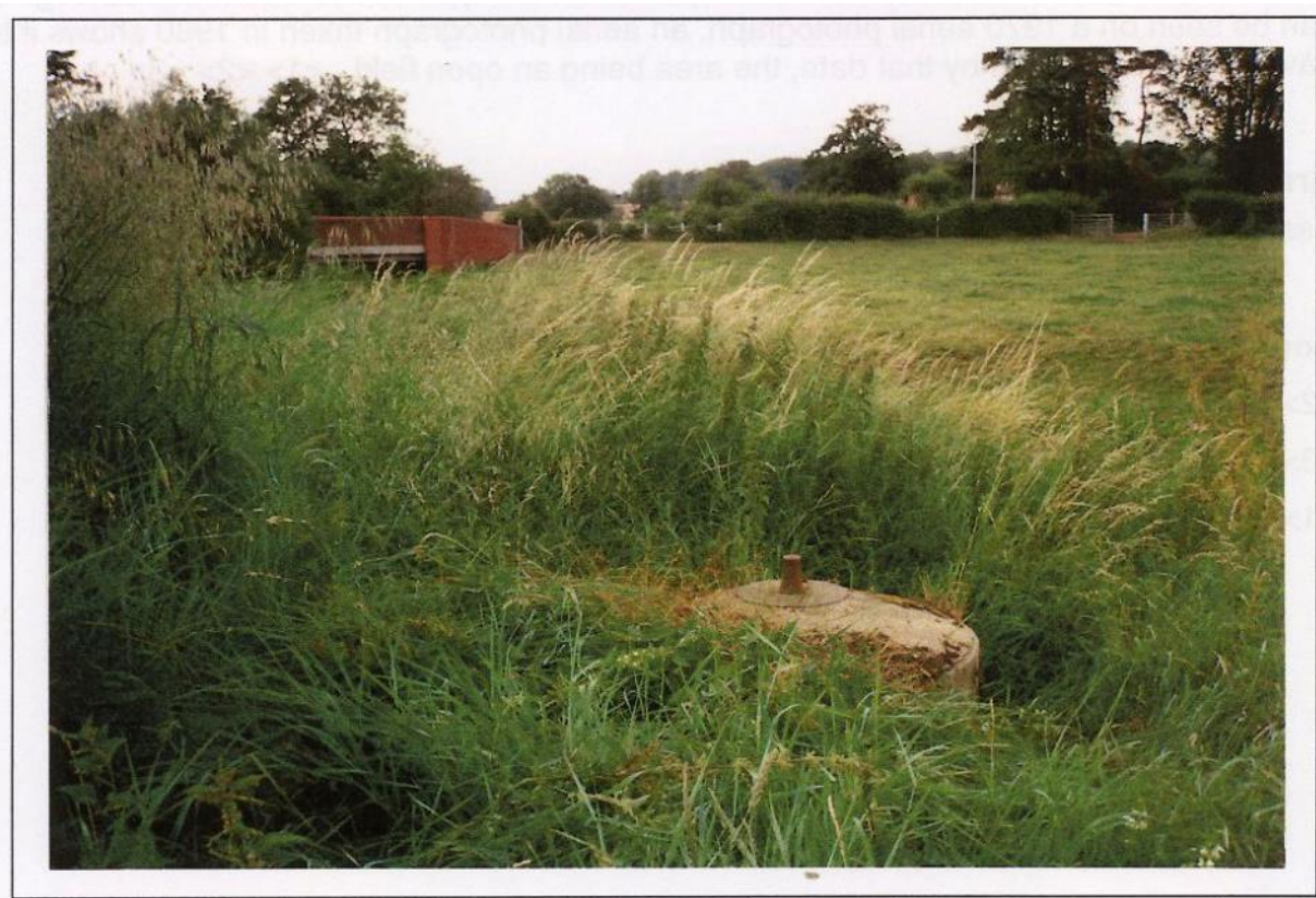
SMR 10950: With less than 50 extant spigot mortar emplacements recorded in the county so far, it is probable that many more lie hidden in the fields and hedgerows, unrecognised for what they are.
