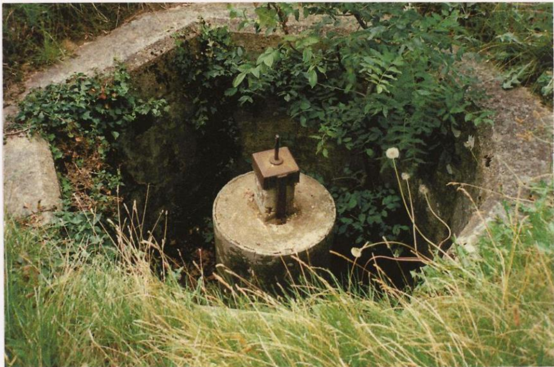
SMR 10957. The anti-aircraft machine-gun well of the Argents Lane pillbox. The pin on the top of the mounting would have held a World War One Lewis gun.
