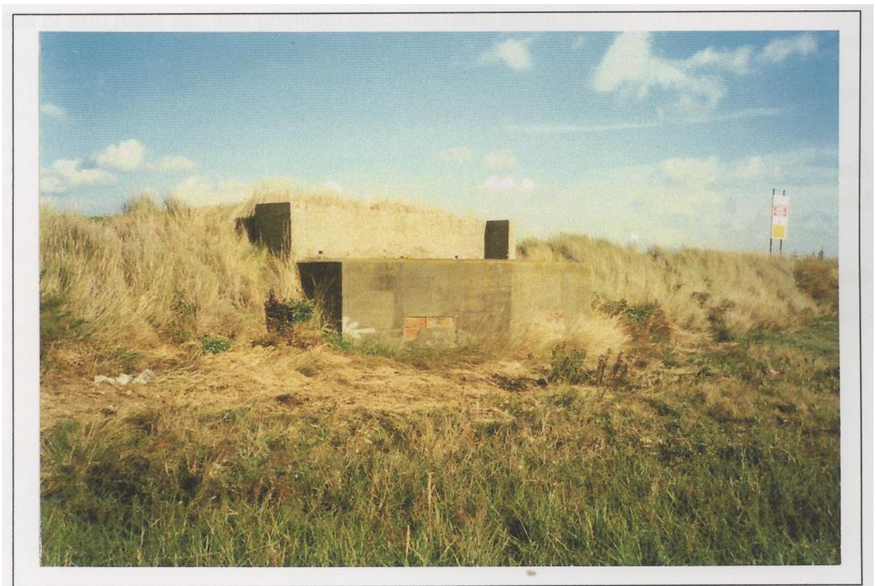
SMR 10733: The loopholes have been sealed since the end of the war to prevent flooding by the sea.
