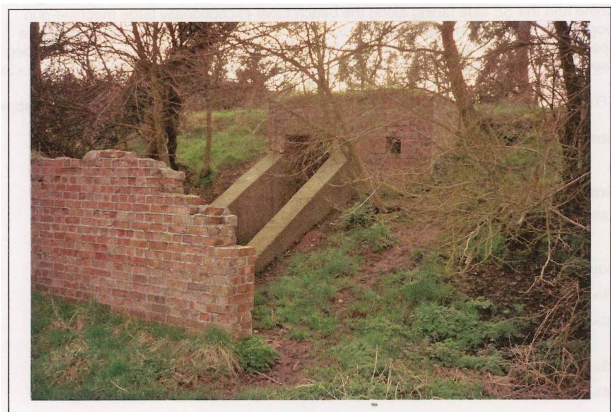
SMR 10036: Pictured in 1993, the decoy bombing bunker at East Mersea has now lost its blast wall.
