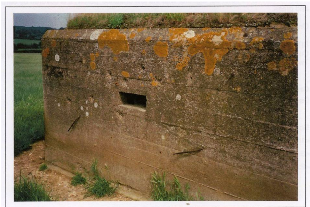
SMR 10962: The hooks, more usually found around the top of a pillbox, were probably to hang camouflage netting
