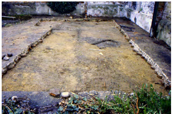
BV96-05-037. SW corner of site immediately after removing concrete. Looking South
